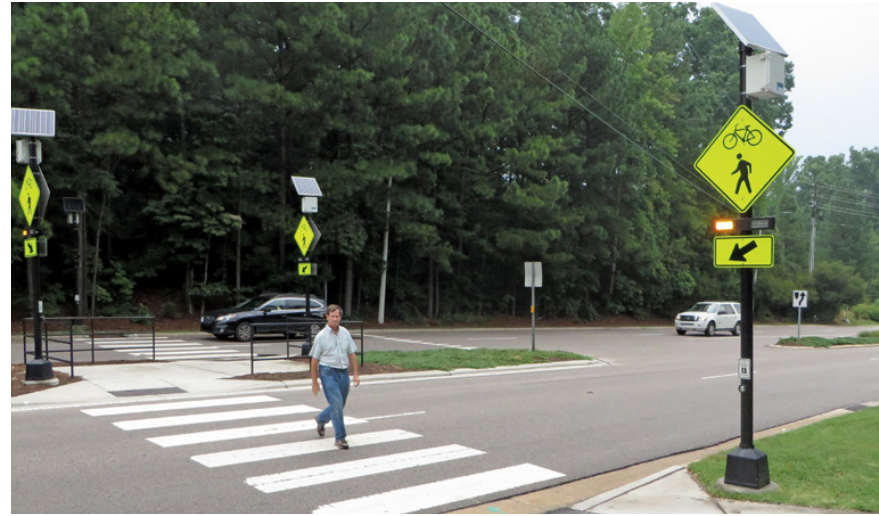
PIANO KEY CROSSWALK WITH RECTANGULAR RAPID FLASHING BEACONS
