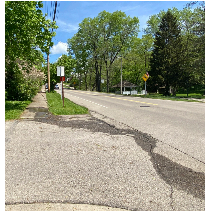
G. NO ADA WARNING MAT AT CROSSWALK
