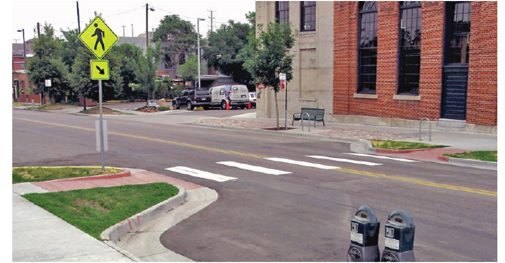
NARROWED ROAD FOR TRAFFIC CALMING
