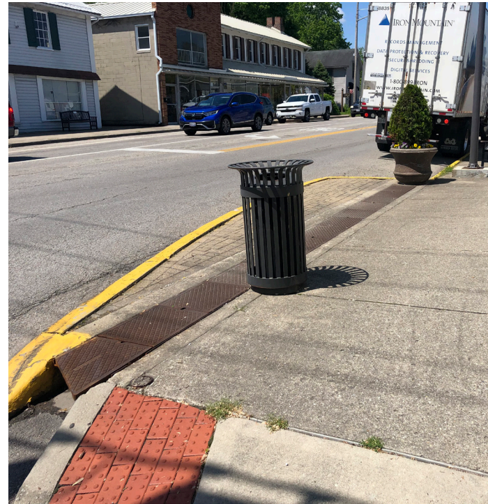
B. STORMWATER CHANNLED TO CROSSWALK
