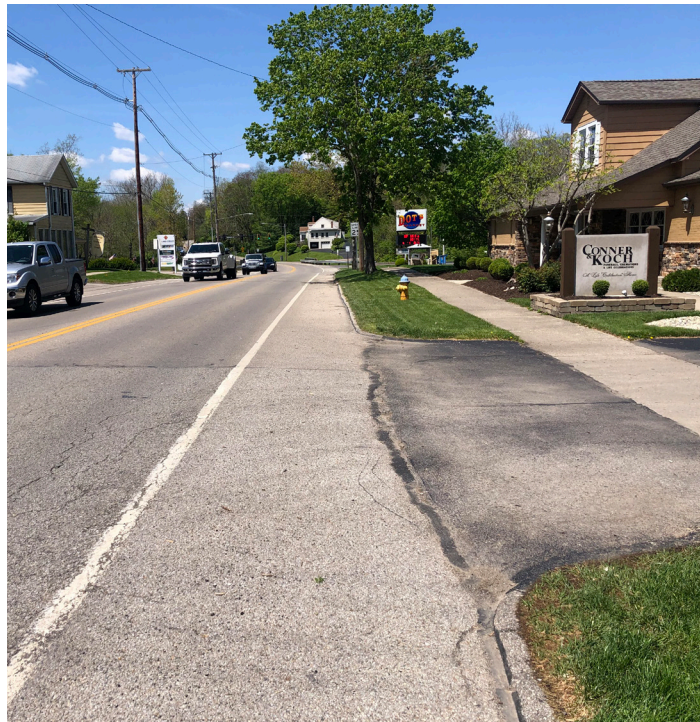
E. UNMARKED BIKE LANE (NO SHARROWS)
