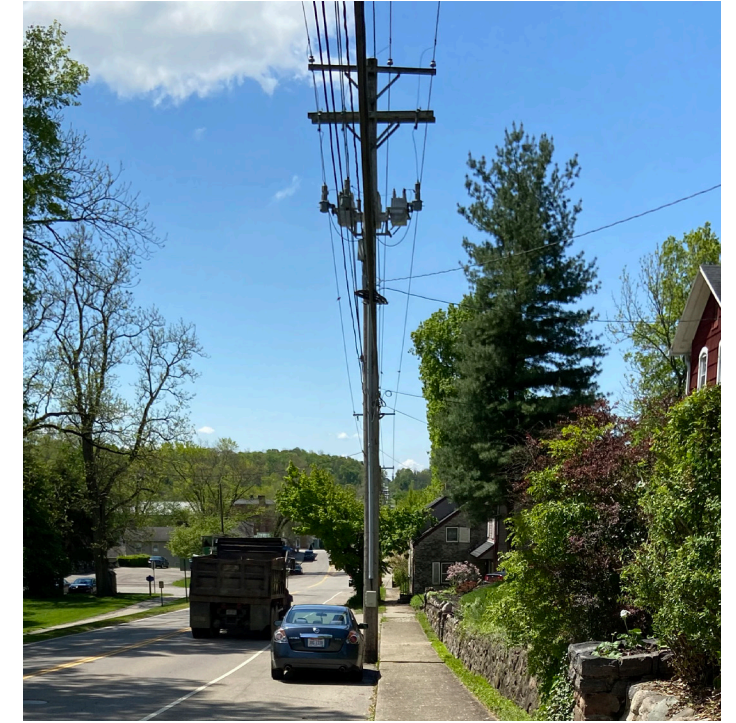
D. UTILITY POLE IN A PARKING SPACE
