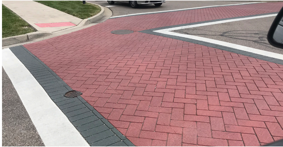
STAMPED ASPHALT CROSSWALK
