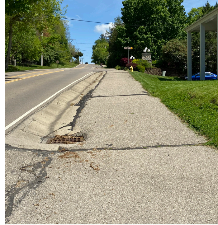
C. STORMWATER CONCRETE FLUME
