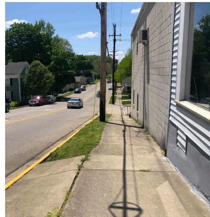
G. OVERHEAD UTILITIES PREVENT PLANTING STREET TREES
