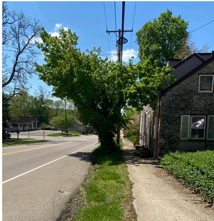
E. TREE TOO LARGE FOR ITS PLANTING LOCATION
