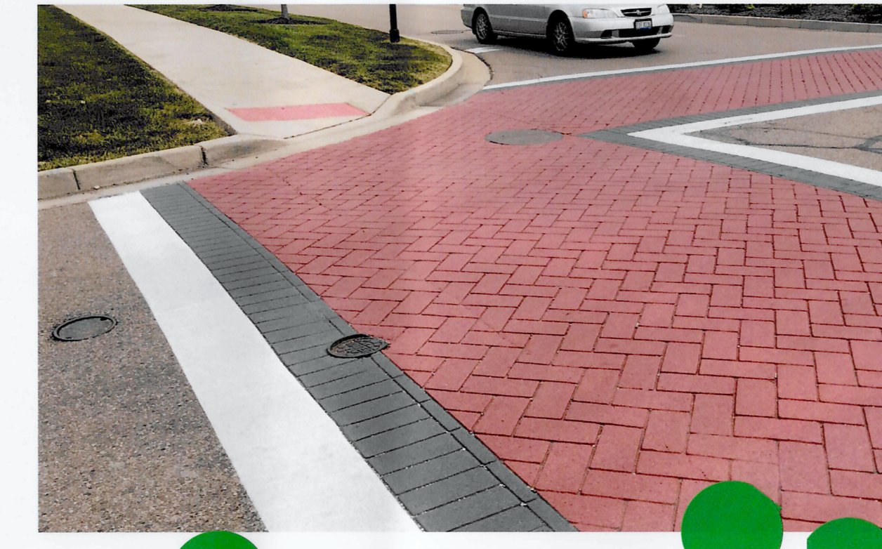
STAMPED ASPHALT CROSSWALK
