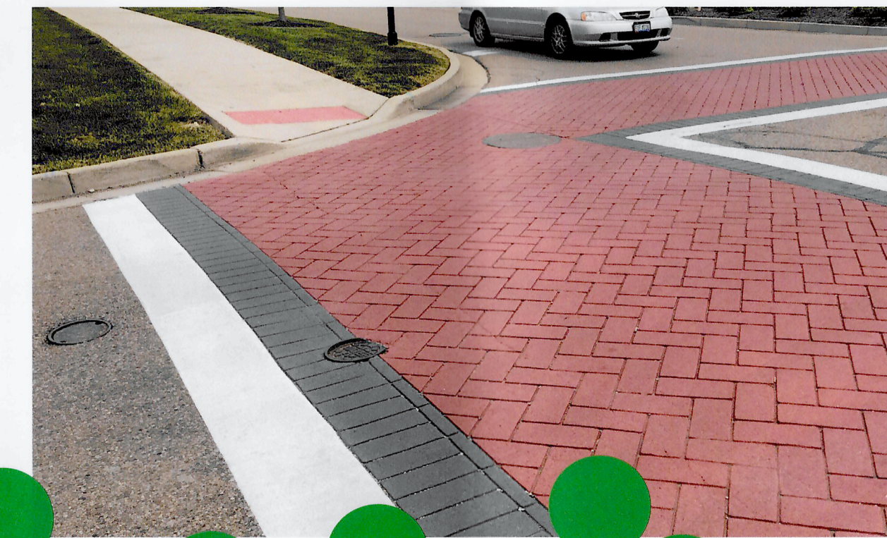
STREET CORNER ASPHALT CROSSWALK AND BRICK PAVERS
