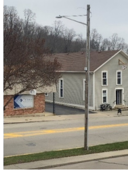
Figure 5: Current light fixtures to be replaced
