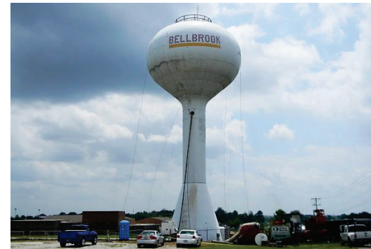
Pictured above: Contractors repainting the Upper Bellbrook Road water tower
