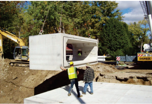
Pictured Below: Contractors working on the Plantation Trail Culvert project
