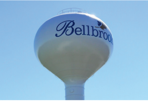
Pictured above: the newly painted Upper Bellbrook Road water tower
