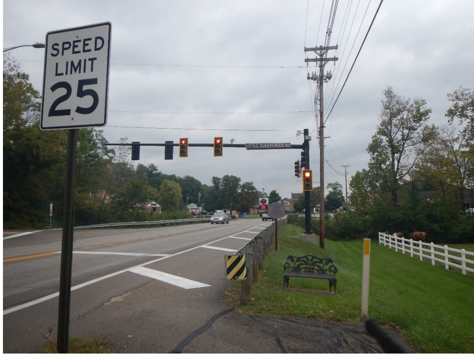
SR725 looking east along bridge
