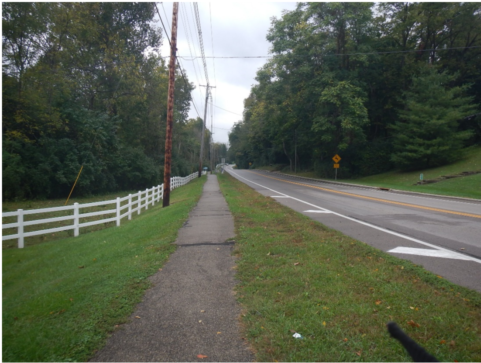
SR725 looking west from bridge
