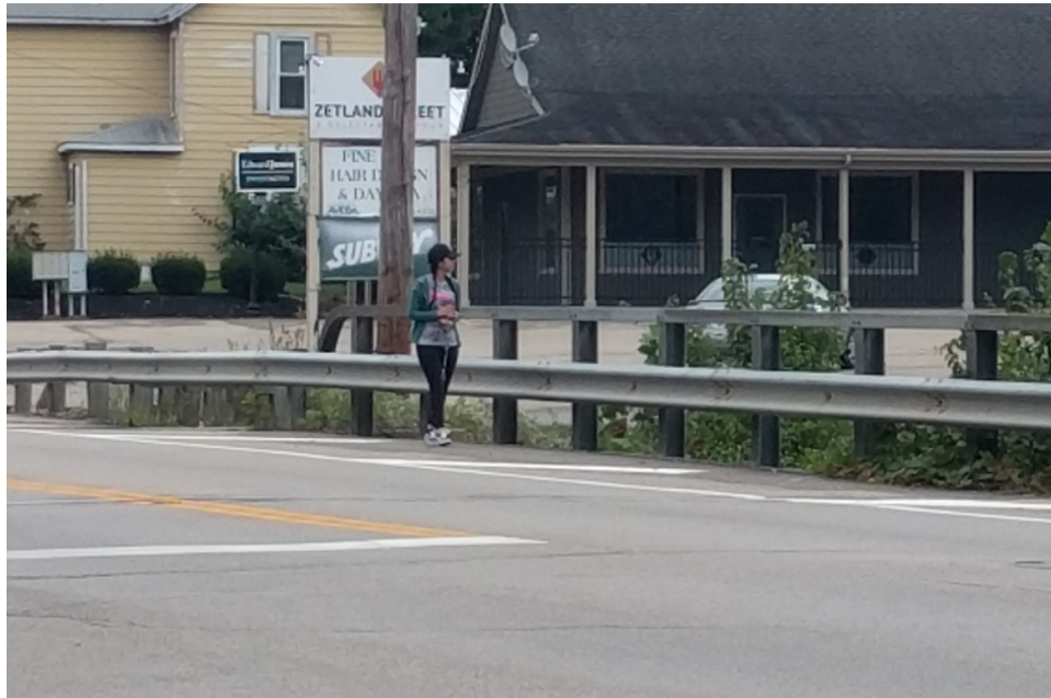
Pedestrian walking along shoulder over SR725 bridge
