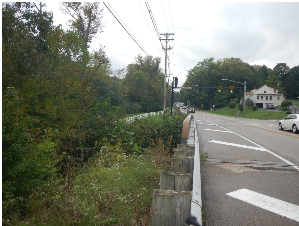
SR725 looking west along bridge
