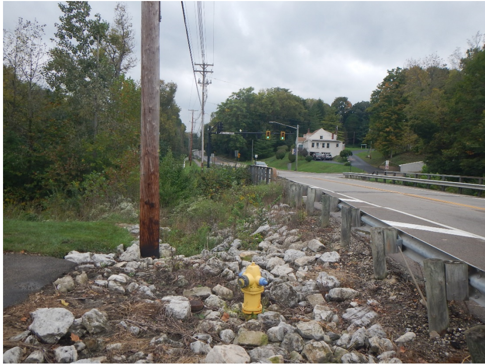
SR725 looking west at bridge
