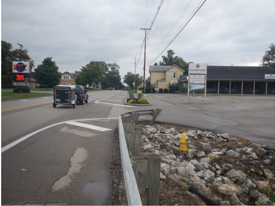
SR725 looking east from bridge
