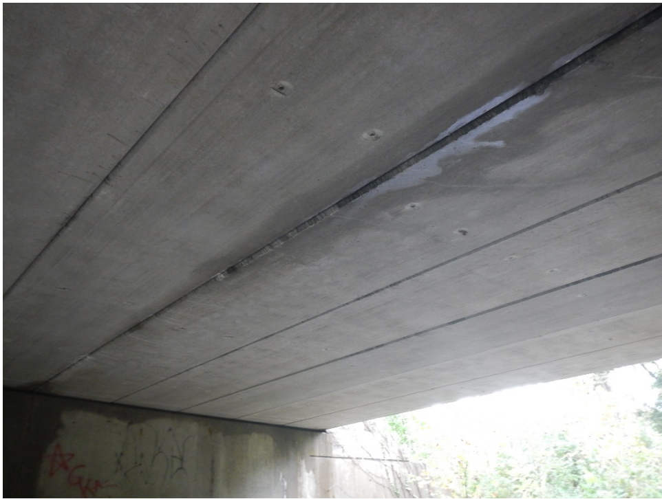
Underneath bridge photo showing prestressed concrete box beams
